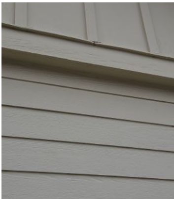
Gap between soffit and fascia
