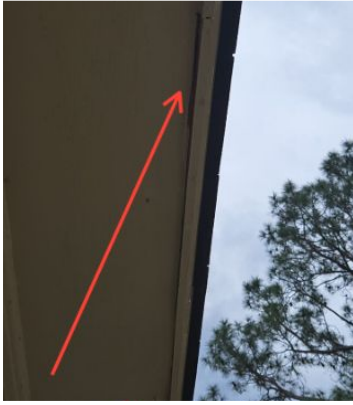
Gap between soffit and fascia
